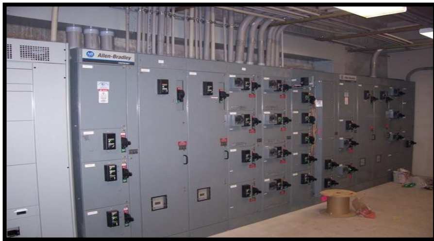
Figure 26: Motor Control Centre (MCC)
