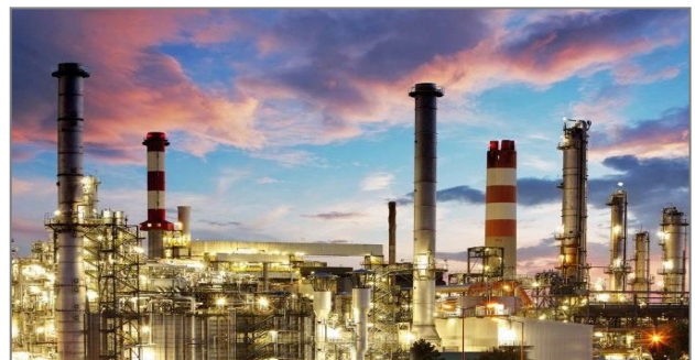
Figure 2: Oil Refinery Process Plant
