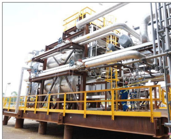
Figure 14: Equipment Structural Support
