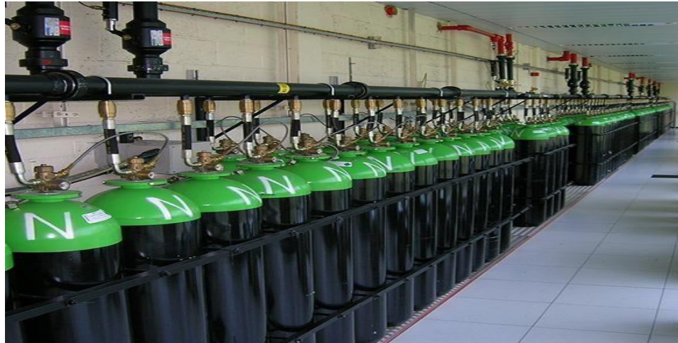
Figure 47: Gaseous Fire Suppression: Inert Gases
