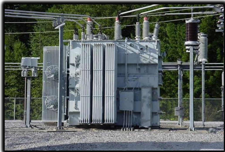
Figure 17: Step-Up Transformer
