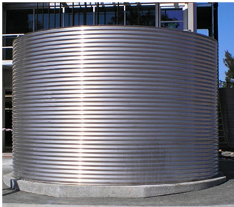
Figure 10: Corrugated Iron Water Tank
