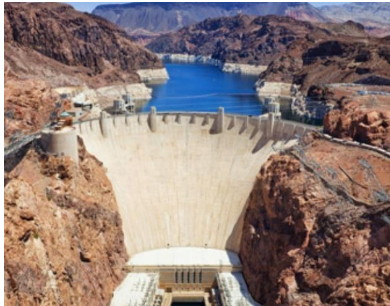
Figure 23: Mass Concrete Dam
