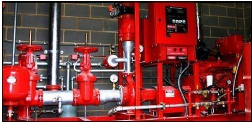
Figure 49: Example of Firefighting Systems (Parallel-Connected Pumps)
